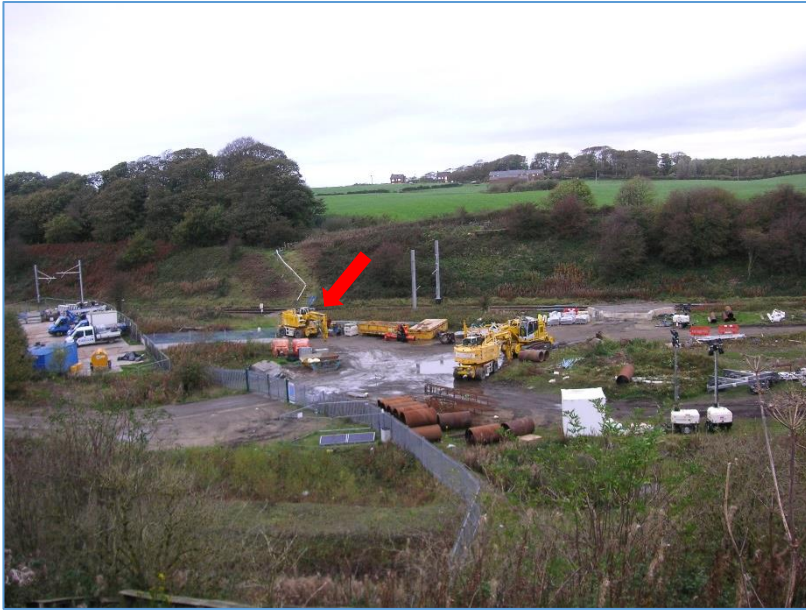
1) From top of embankment on south side of railway site. Red arrow marks location of Kirkham Tip Level Crossing.
