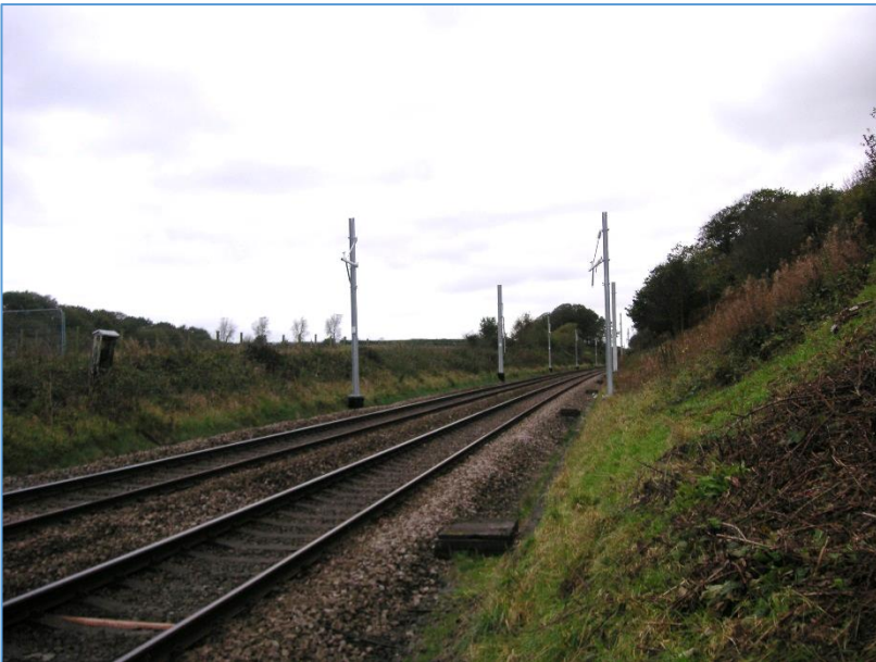
5) From point B at north side of railway, looking west.
