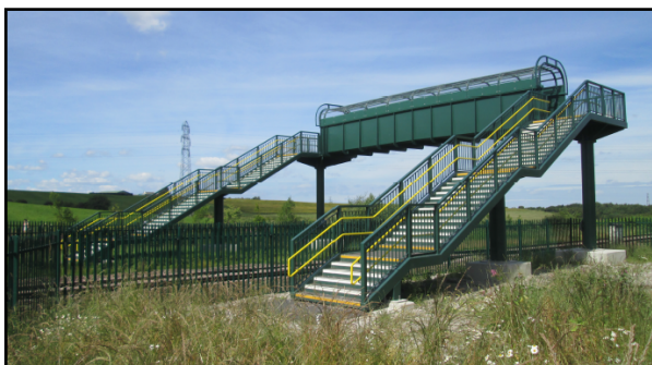
Figure 1: An example of a stepped structure
