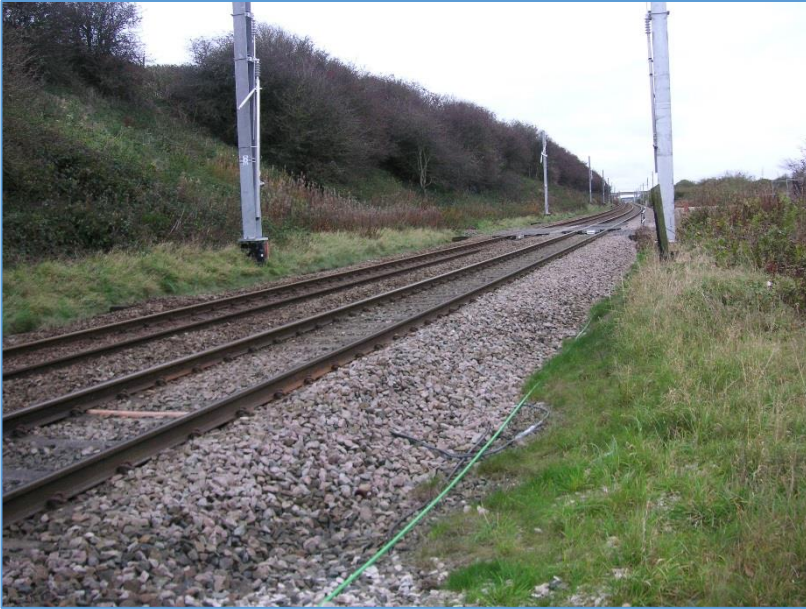
4) Looking east from south side of railway.
